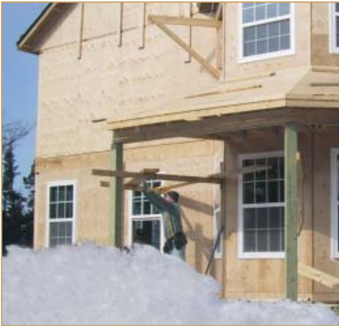
Credit: Ronalda Steele Construction work underway in Paradise
