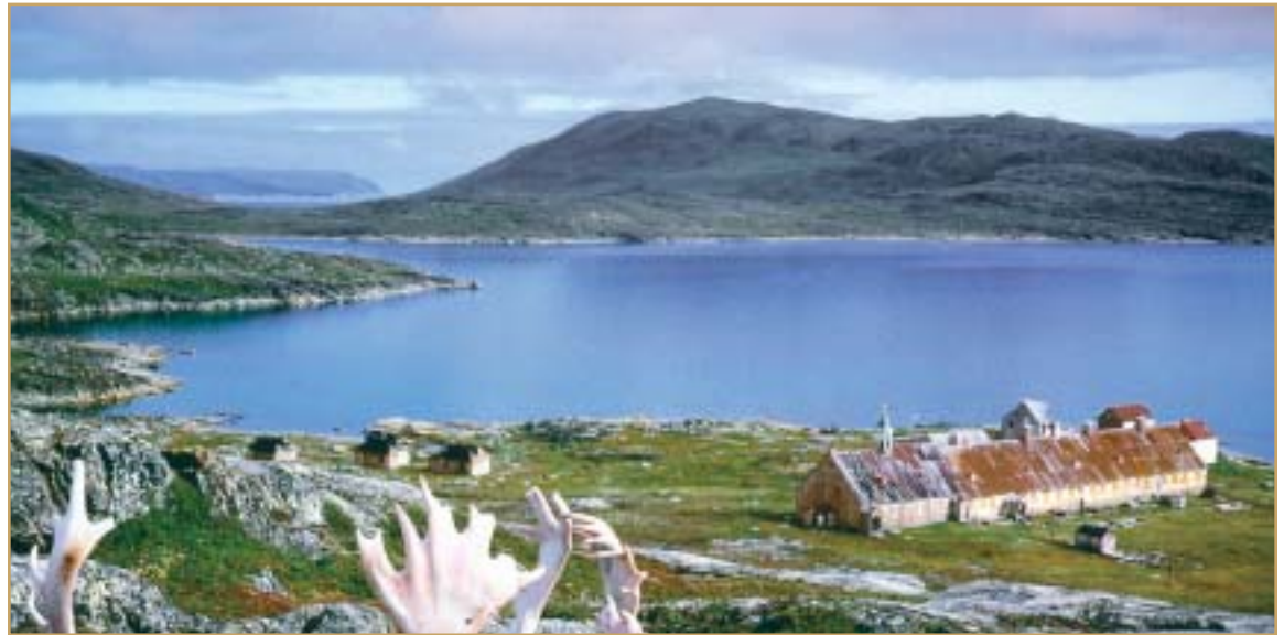
Credit: Department of Tourism, Culture and Recreation The Moravian Mission at Hebron Bay, Labrador is one of the oldest surviving man-made structures in eastern Canada
