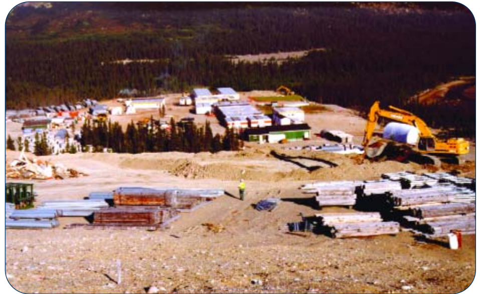
Credit: Voisey's Bay Nickel Company Limited Voisey's Bay construction site.
